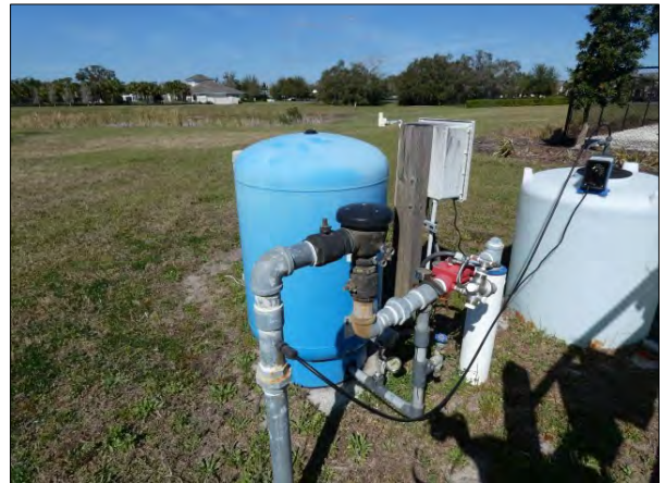
Well and Pressure Tank
