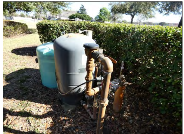
Well and Pressure Tank
