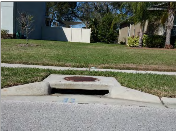
Stormwater Drainage Curb Inlet
