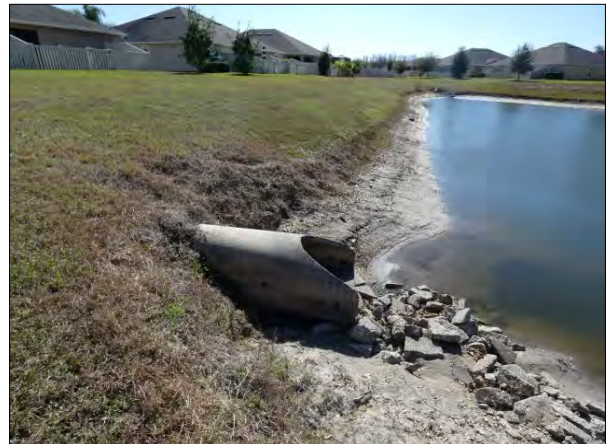
Stormwater Drainage Mitered End Section
