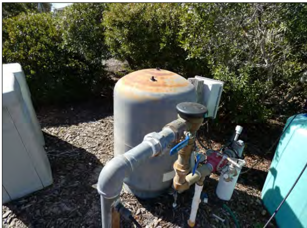
Well and Pressure Tank
